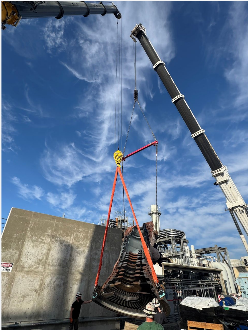
Steam Turbine Top-Case Flip
